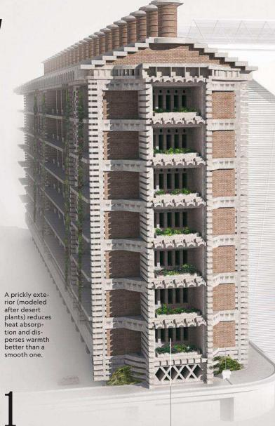
Double-thick brick walls and precast concrete have high "thermal masses"; it takes a lot of heat to change their temperatures. The same is true of soil around termite nests.
